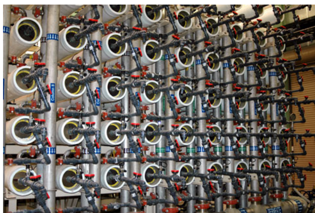
Fig. 3 Reverse osmosis water treatment plant at Bingham Canyon, UT, USA
